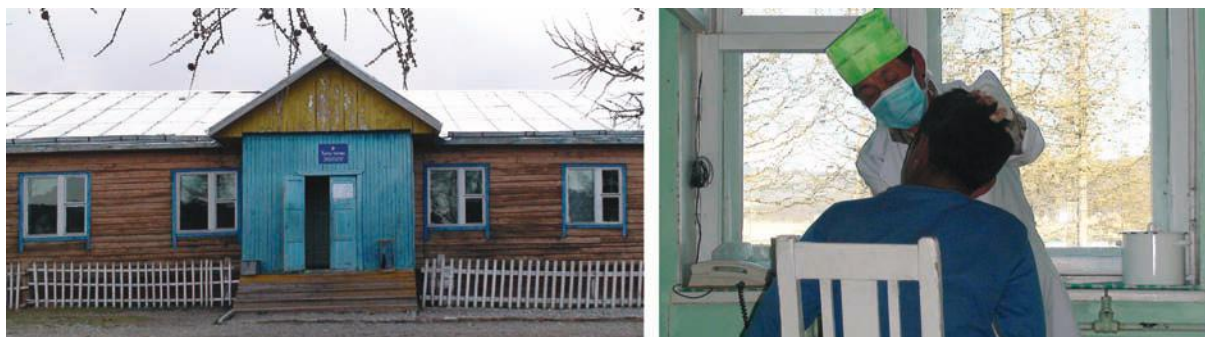
Figure 49-17. First Level (Soum) Hospital. (Photos reproduced with permission from Raymond R. Price MD. Layout reproduced with permission from Intermountain Healthcare.)
